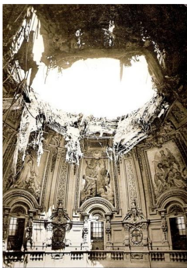
Photo 9. Wartime damage showing the destruction of the main dome
