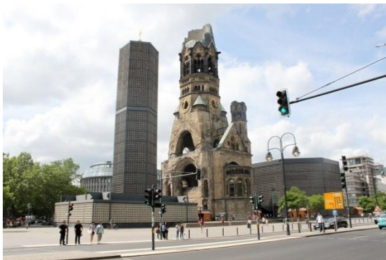
Photo 13. The new elements around the remains of the ruin
