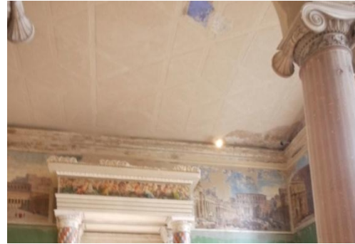
Photo 19. Damaged wall frescos stabilised ‘as found’
