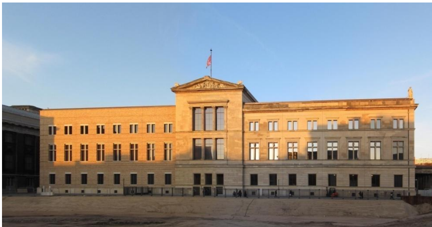
Photo 6. The restored façade in 2009, with the façade to the left reconstructed without its classical ornamentation
