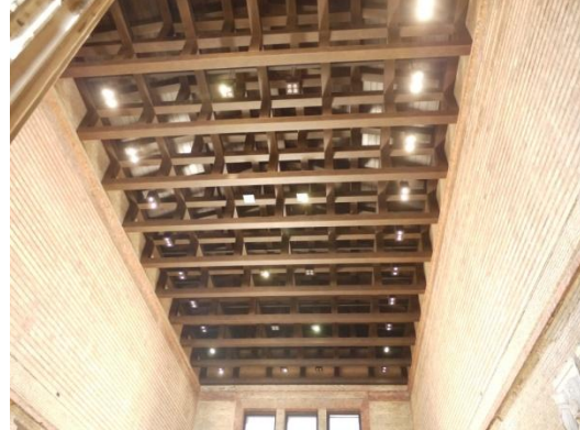
Photo 23. A visually oppressive new roof structure
